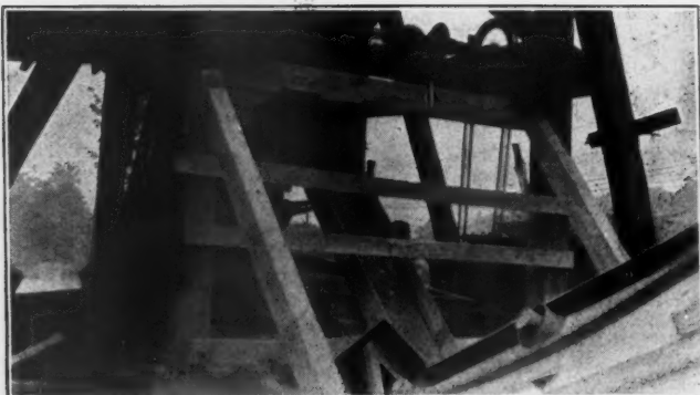
Chute and Conveyor Which Carries Gravel from Screen to Bins Nature of Deposit. Crane is Used for Stripping
